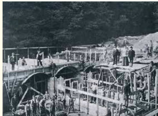
Bau eines Wasserreservoirs in Eisenberg, 1884 Construction of a water reservoir in Eisenberg, 1884
